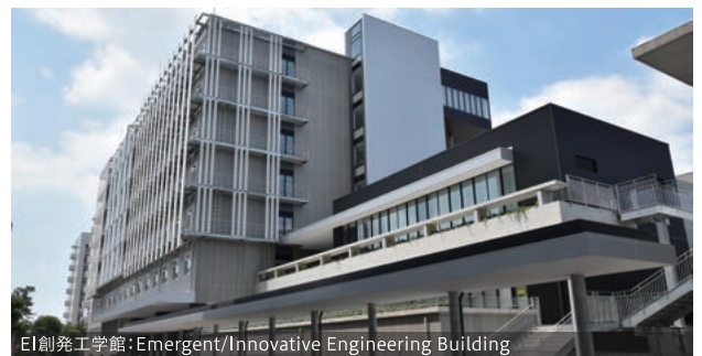
EI創発工学館: Emergent/Innovative Engineering Building
