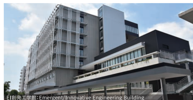
EI創発工学館: Emergent/Innovative Engineering Building
